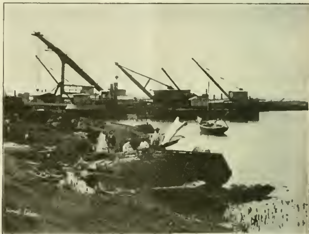
CANAL DREDGES—FOX RIVER, NEAR COLON.
